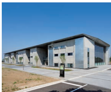
Research and Testing Complex I, Institute of Industrial Science (IIS)
